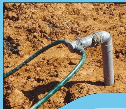
FIGURE 27. Hydrant of low-pressure pipe system with flexible hose connections
