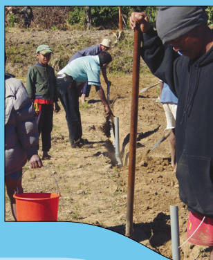
FIGURE 28. Installation of low pressure pipe system – SPFS in Madagascar
