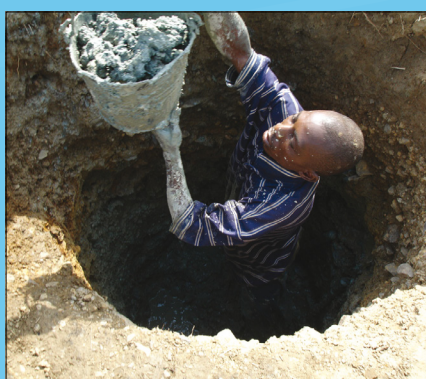
FIGURE 3. Open well development and lining with concrete rings – SPFS in Sierra Leone
