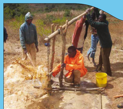
FIGURE 4. Training of drilling team in rota sludge technology for well development – Practica Foundation
