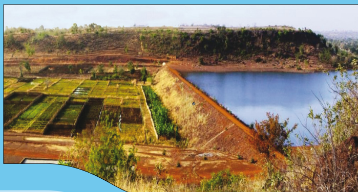
FIGURE 7. Small earth dam for irrigation – Burkina Faso (from GRAF-B.W. Sanou)
